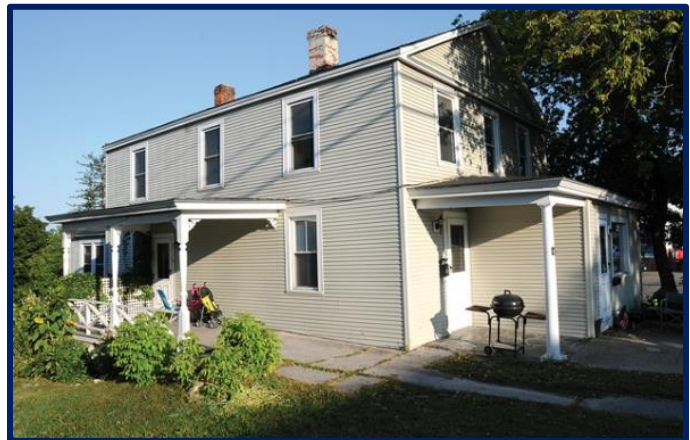
A Vermont multi-family house which received weatherization assistance. Source: Vermont Energy Investment Corporation.
