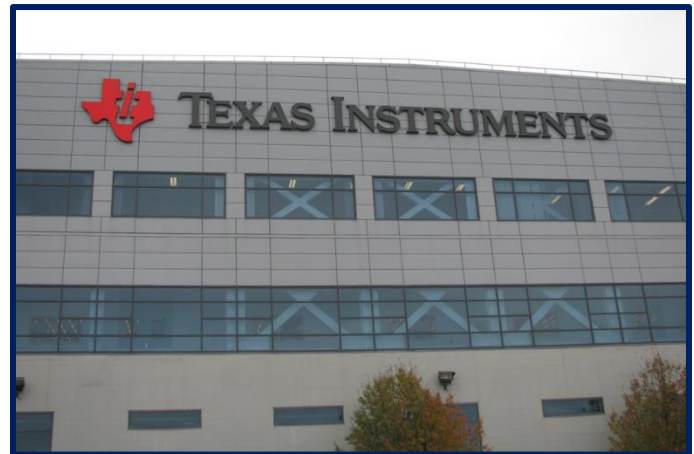
Texas Instruments' South Portland, Maine wafer fabrication facility. Photo Courtesy of Texas Instruments
