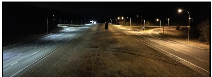
I-295 Exit 7 – Smithfield, during the process of converting to efficient LED lighting. The left side of the highway are LEDs. Source: RI Office of Energy Resources.
